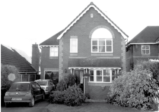
25 Vaughan Road, Cleobury Mortimer £225,000 Detached house • Four Bedrooms • Single garage Oil fired central heating • Security alarm
